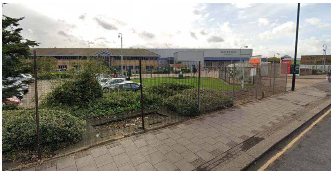
Figure 4: Existing poor streetscape along Southbury Road
